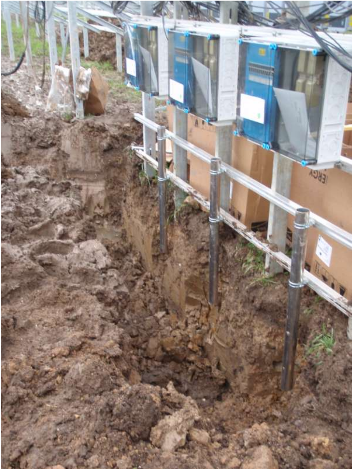
Plate 3. View showing hand digging to connect switchgear (Phase 1)
