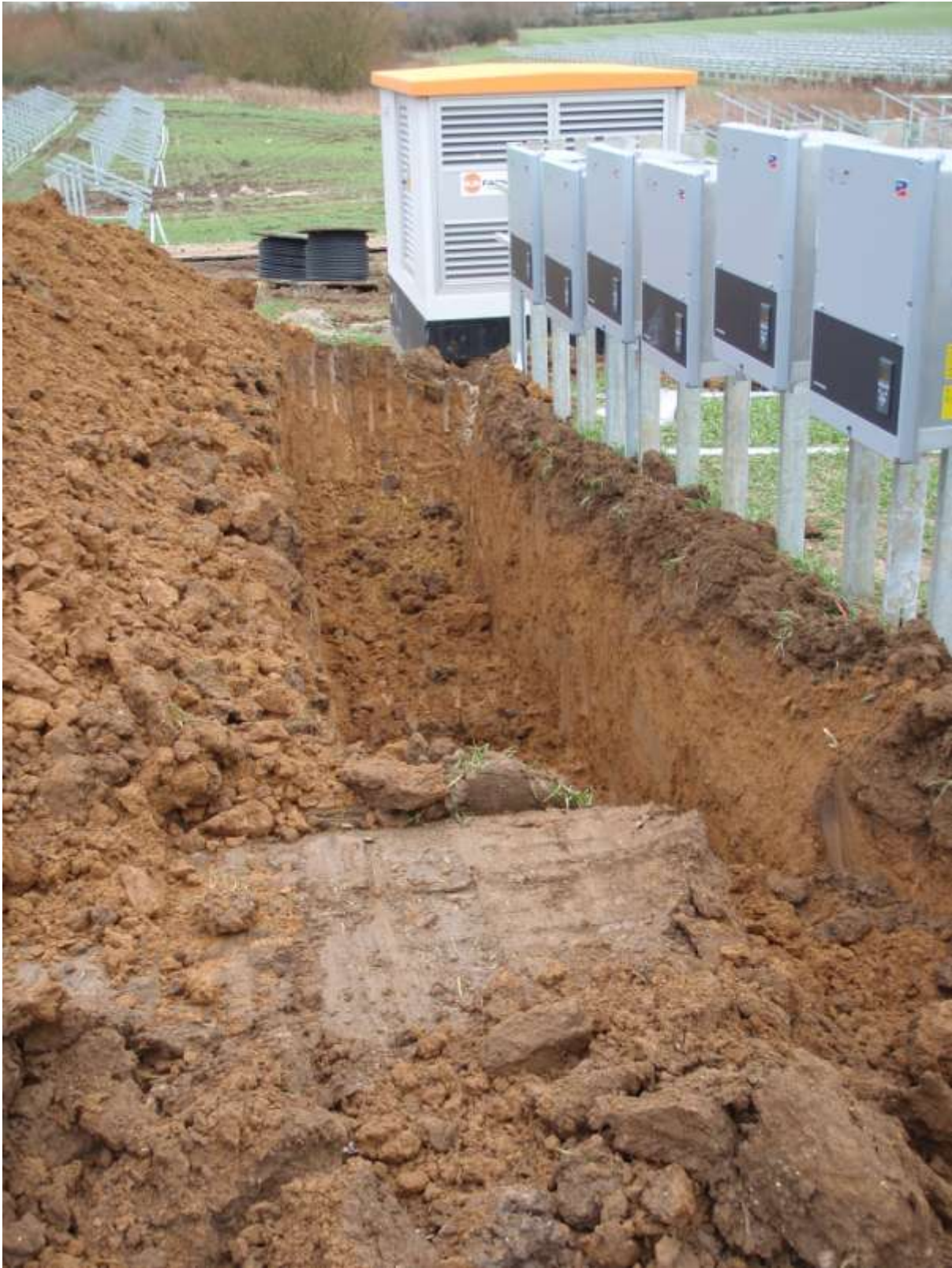
Plate 4. The site showing invertor and switch gear (Phase 3)
