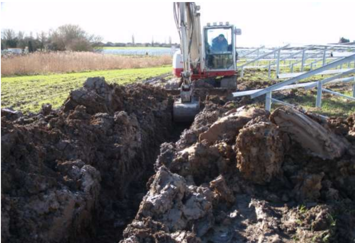
Plate 8. View of cable trench array connections (Phase 4)
