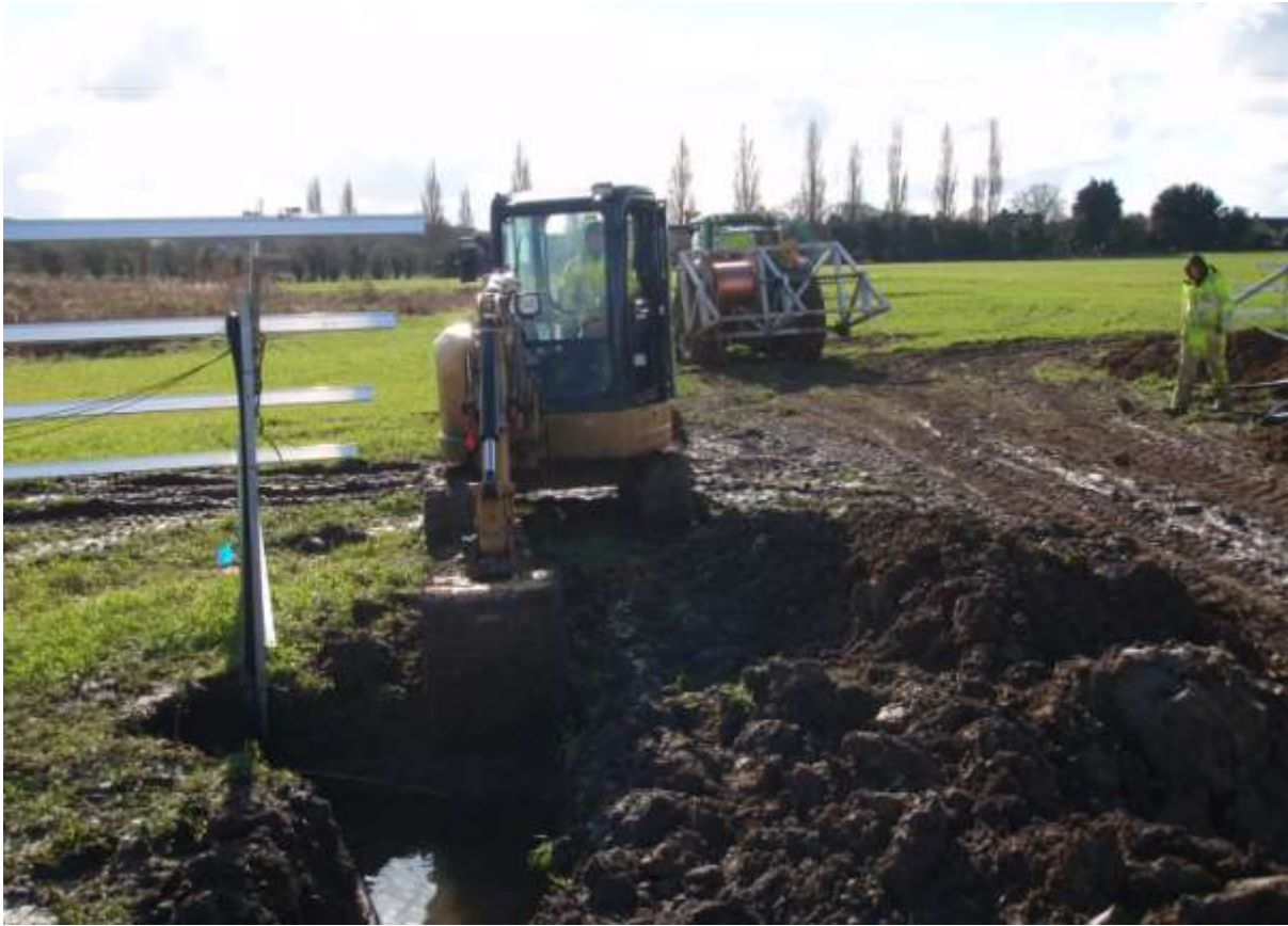
Plate 7. View of cable trench array connections (Phase 4)
