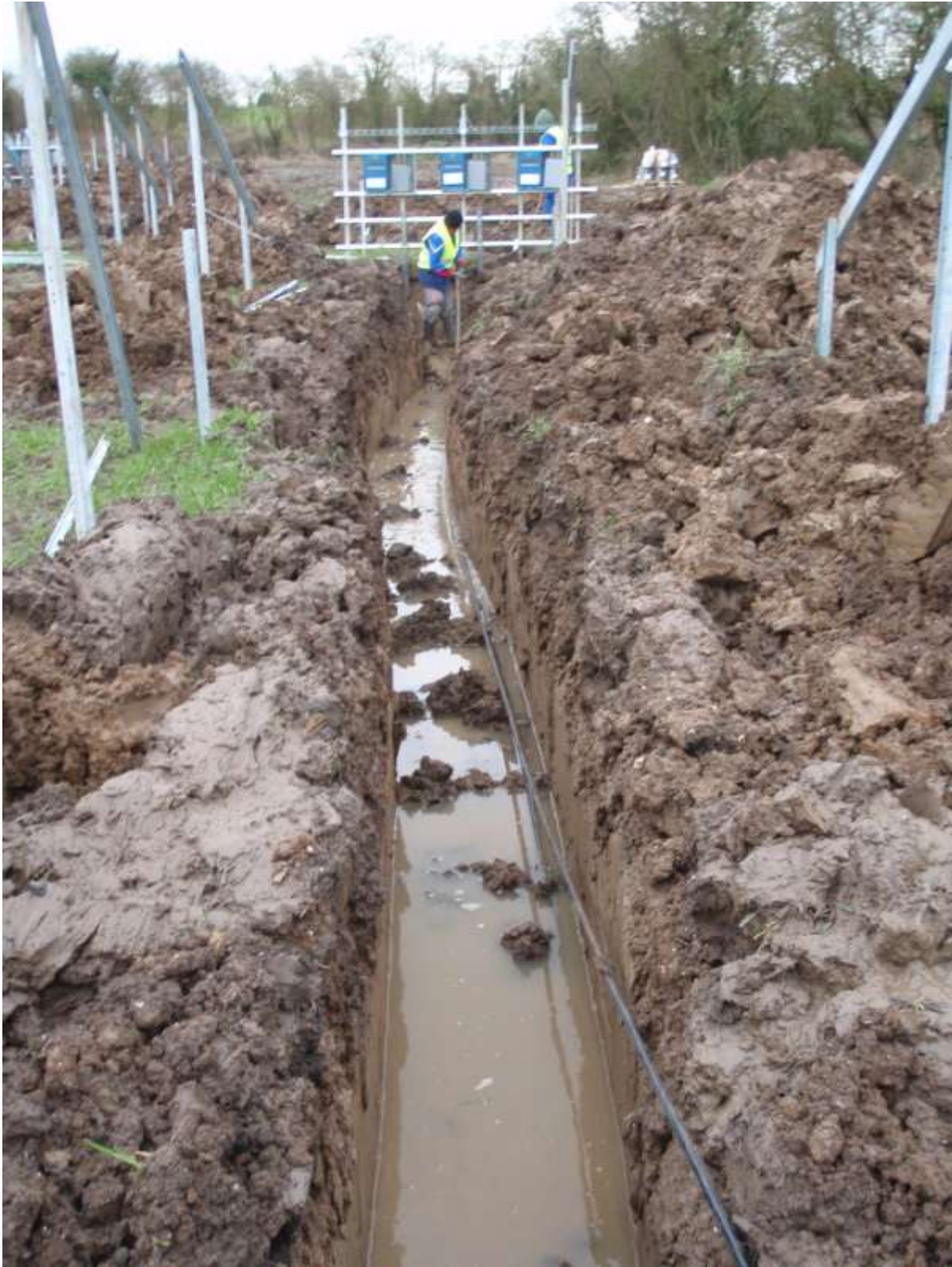
Plate 2. View of trench for switchgear (Phase 1)
