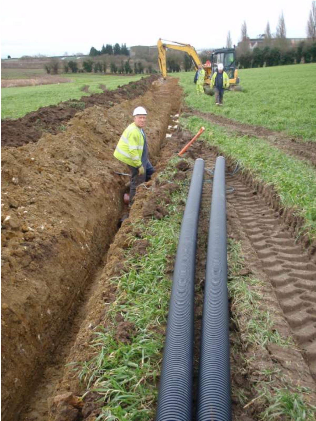
Plate 5. View of connection cables in quarried brickearth backfill (Phase 2)
