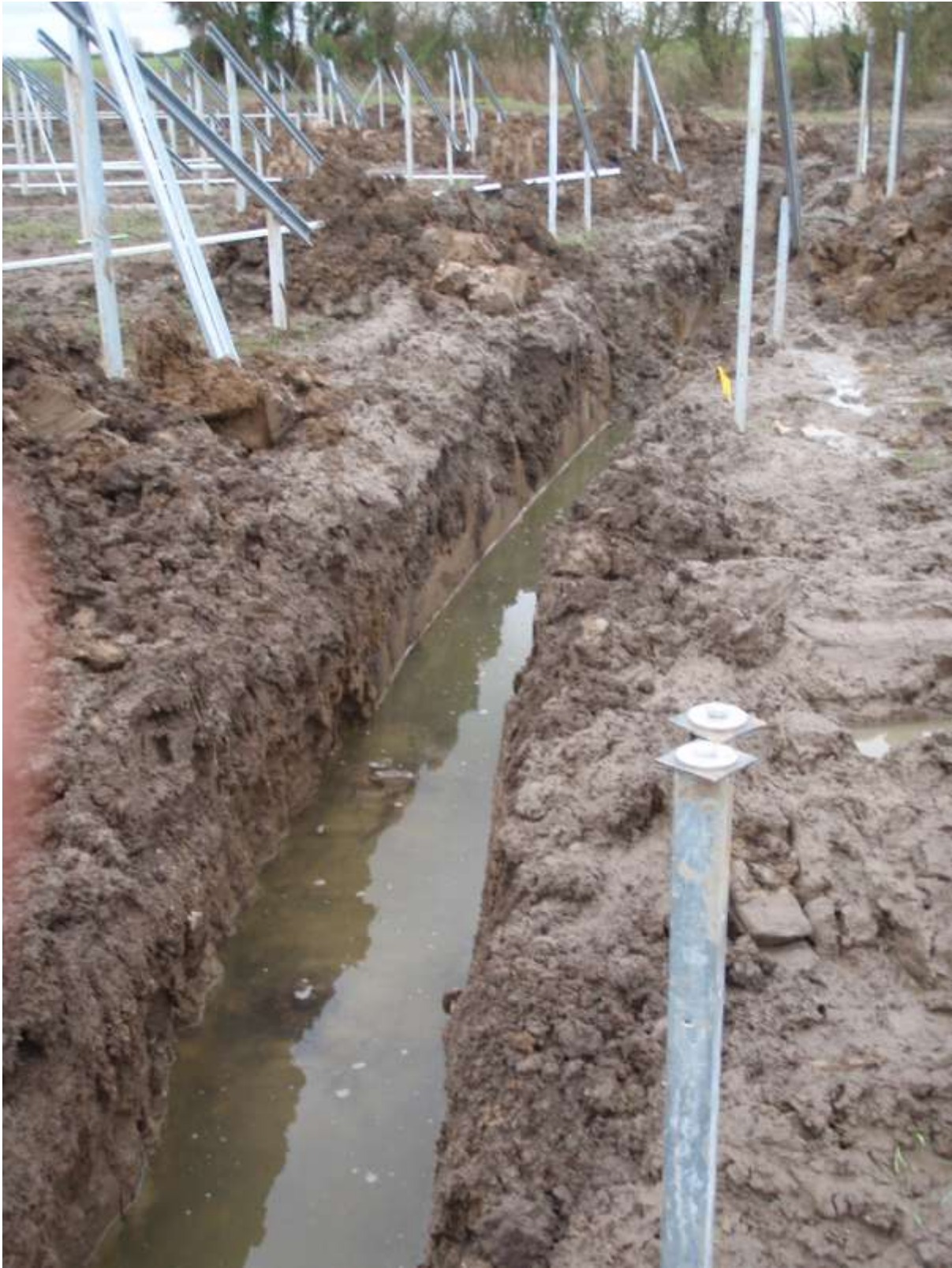
Plate 6. View of cable trench array connections (Phase 4)
